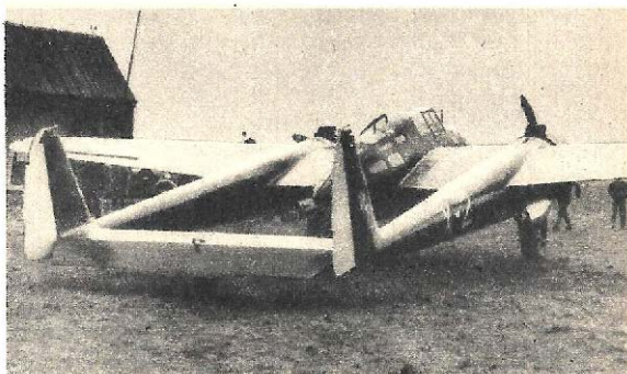
This Fokker G-1 combination combat-pursuit-bomber airplane was built for the Dutch Air Force. The fuselage rear end (between the two tails) features a revolving gun turret.
