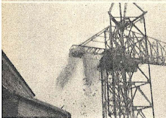
When it was necessary to remove a massive reinforced counterweight from a marine crane, dynamite was used. A camera caught the actual blast. The steel work was not damaged. —Photos Courtesy E. I. du Pont de Nemours & Co.
