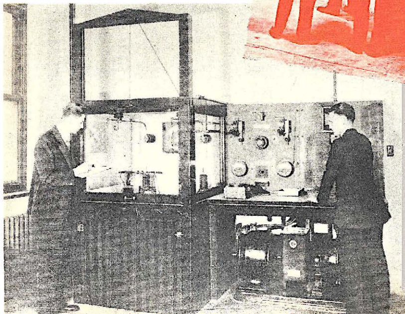
Above—A made-to-order "standard fire" is used to test the qualities of a fire window. The window is subjected to extreme heat and water under a 35-pound pressure.
