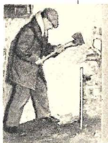
Examples of good grounds. Long pipes driven through the wall or floor are one of the best forms of ground for the average radio fan. When a well or cistern is available, a good connection may be made at these points. In all cases be sure the actual connection points are bright and clean.
