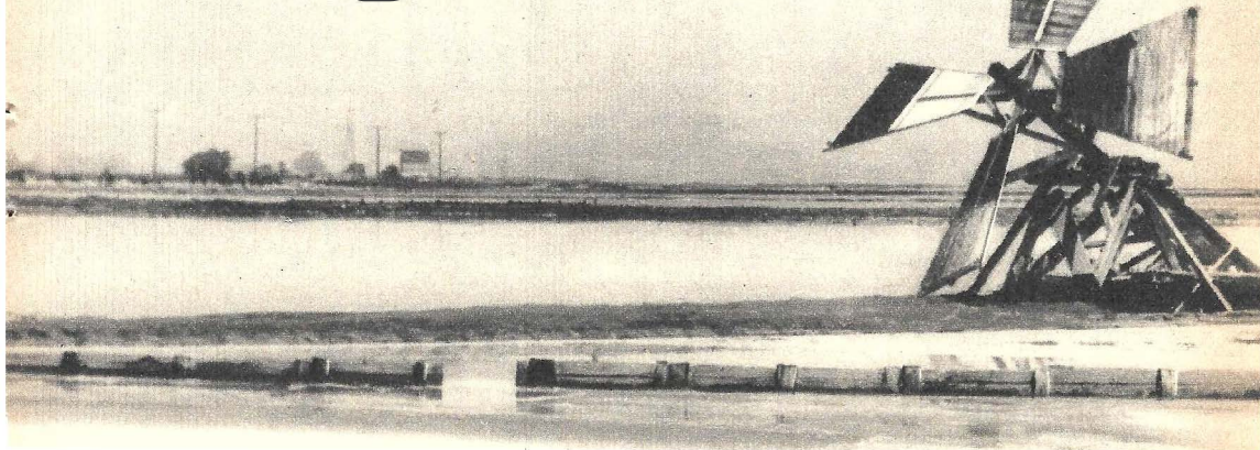
A relic of the early days of the Alvarado Salt Farms. Called the Archimedian windmill, it received its name because the ancient Greek mathematician Archimedes is credited with being the first person to construct a windmill for pumping water.
