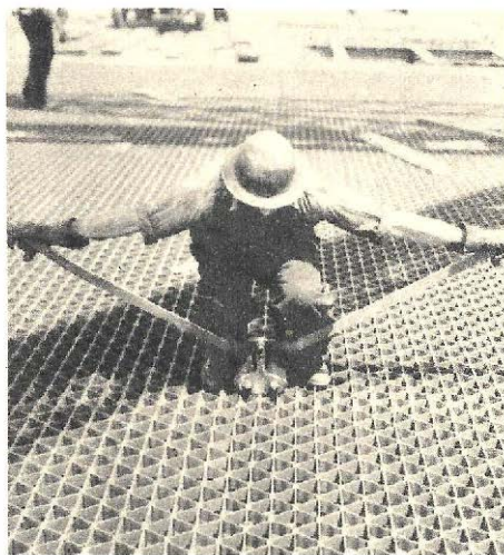
This worker is bolting together a section of the fabricated steel grillwork that is being used as the roadway on the Marine Parkway Bridge connecting Brooklyn and Long Island.
