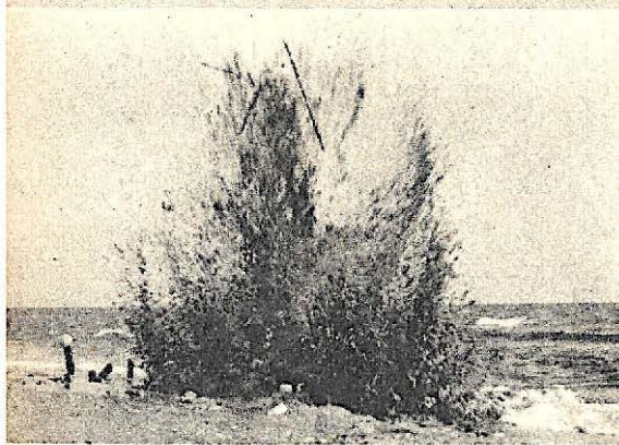
Charges of dynamite in the sand alongside the piling are shot in series by the electrical method of setting off blasts, thus cutting off a number of piles at one time.
