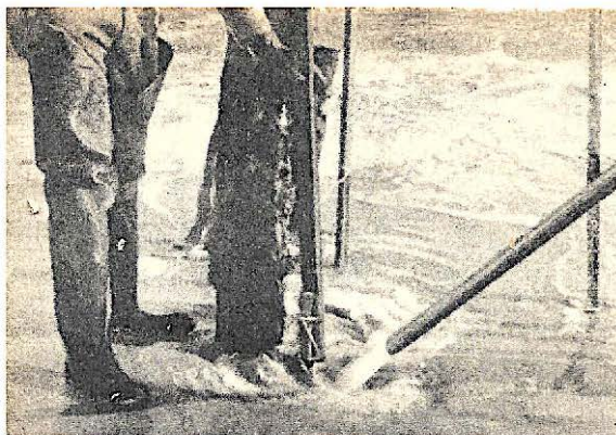
Preparing to remove piling by dynamite. A water jet is used to displace sand, and as the hole alongside the piling is made, dynamite attached to a pole is pushed down into the cavity.
